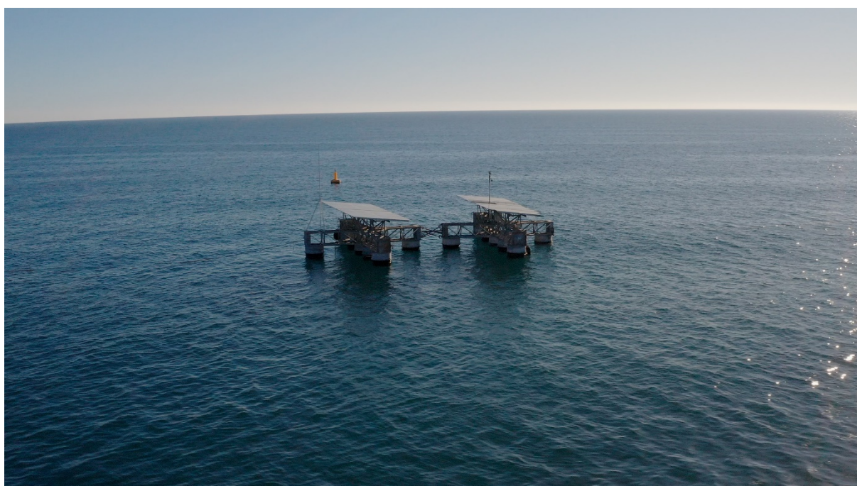
Sun'Sète – First offshore solar farm in the Mediterranean, December 2023
